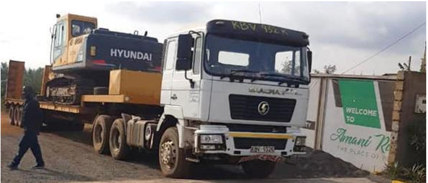
ABOVE: Construction machinery arrives at AMANI RIDGE | The Place of Peace ahead of the revamping and upgrading of road infrastructure at the project on 13 th October 2020
