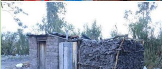
ABOVE: Mama Nduko outside her new house built by Optiven while below is her old house before the intervention.
