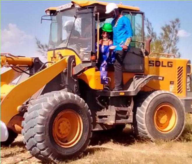
ABOVE: Dr. Jones and Dr. Mrs. Beatrice Lukose, both Kenyans resident in the Netherlands aboard a digger on 17 th March 2022. The event was a ground breaking for their home at Victory Gardens
