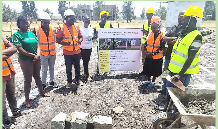
ABOVE: The Optiven team joins engineers and architects from Bejoy Enterprises Limited during a ground-breaking ceremony for a customer at Victory Gardens in Kitengela in January 2026.
